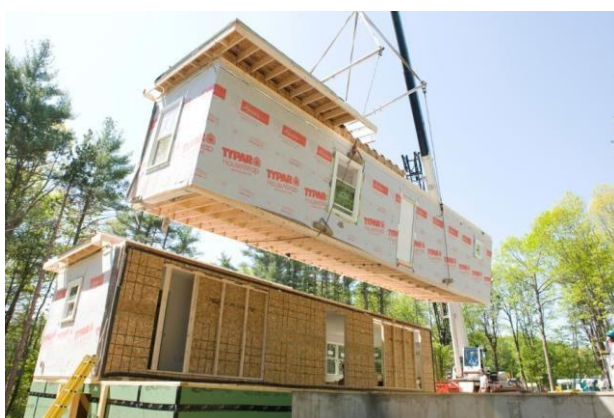
Figure 2. (b) Volumetric prefabs Source: Solymári, et al. (2021).
